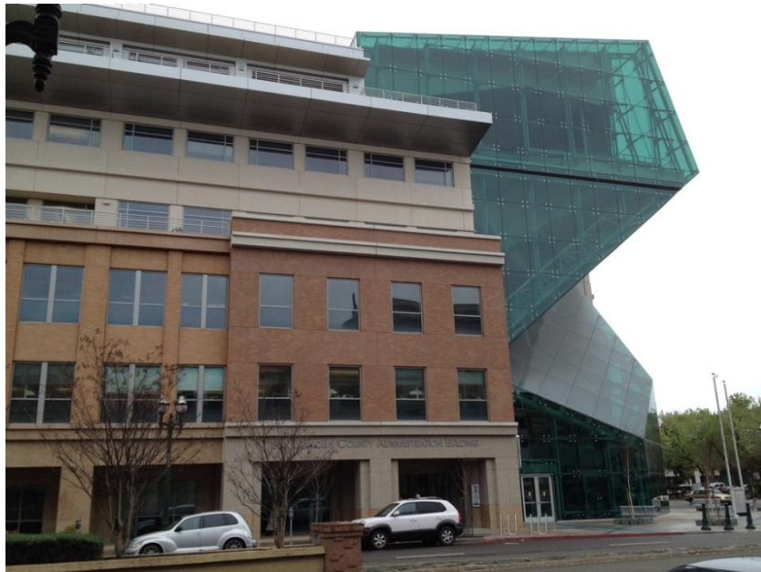
New county building directly across the street
